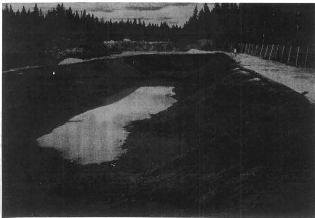
Fig. 12 A pit sealed with Wastolan. It is supposed to be impervious to sewage to avoid seepage and pollution of the soil.
